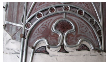
Another window being restored
