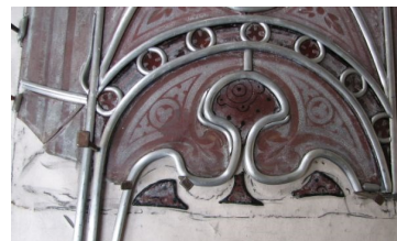
Another window being restored
