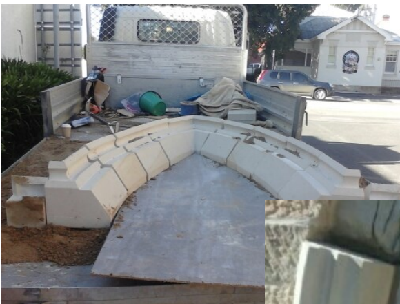
Left: Pieces of an arch for the west windows.
